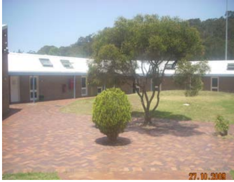
The accommodation at the Retreat venue, Department of Sport and Recreation, Narrabeen
